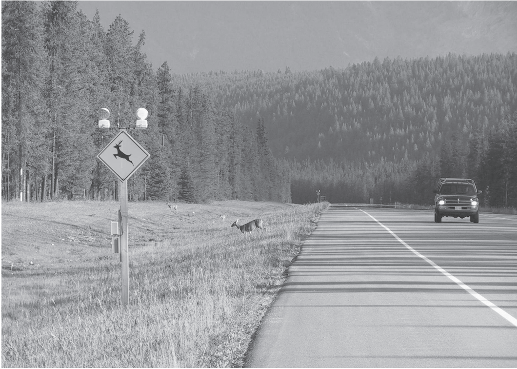
Figure 10. The Wildlife Protection System uses an infrared camera to detect animal presence along roadways, which subsequently triggers flashing lights warning approaching motorists. Highway 93 near Dolly Varden Creek, Kootenay National Park, BC. (Alan Dibb).
